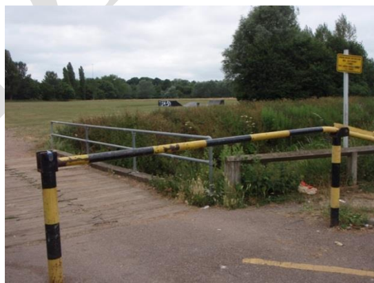
Bridge and barrier at Woolgrove Road car park
