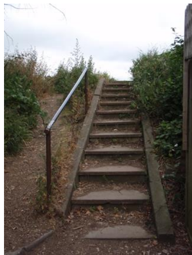
Steps at Common Rise entrance
